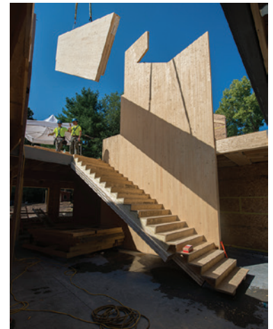
For the $7.5 million, Type VB, 15,000-square-foot addition, the project team chose a combination of CLT and glulam. The new school building was framed in just four weeks by a crew of five, using prefabricated materials. Architecture: Gray Organschi | Photos: David Sundberg
