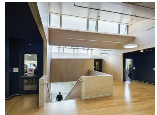
Black spruce CLT panels act as the tension surface and final ceiling finish in a revolutionary system of prefabricated stressed skin assemblies that span the upper classrooms and circulation spaces. Architecture: Gray Organschi | Photos: David Sundberg
