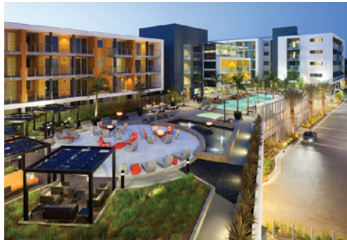
Two things make this project unique: the fact that it includes a Type III building with five stories of wood and a Type V building with four stories of wood on a shared concrete podium and the use of prefabrication to speed the building process. Images courtesy of Lawrence Anderso
