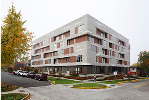
COOL FOR SCHOOL | University House Arena District, Eugene, OR Podium construction can be an efficient and cost-effective way to meet the rapidly growing demand for student housing across the country. This 109,600 square-foot student housing project includes five stories of wood-frame construction over a concrete podium achieving an attractive yet affordable design. PHOTO CREDIT: Lincoln Barbour | ARCHITECT: Mahlum Architects
